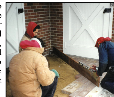
Laying out the bricks, 1996
